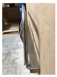
1. Secure the main seat support bar to the wall using the mounting holes in the bracket provided.
